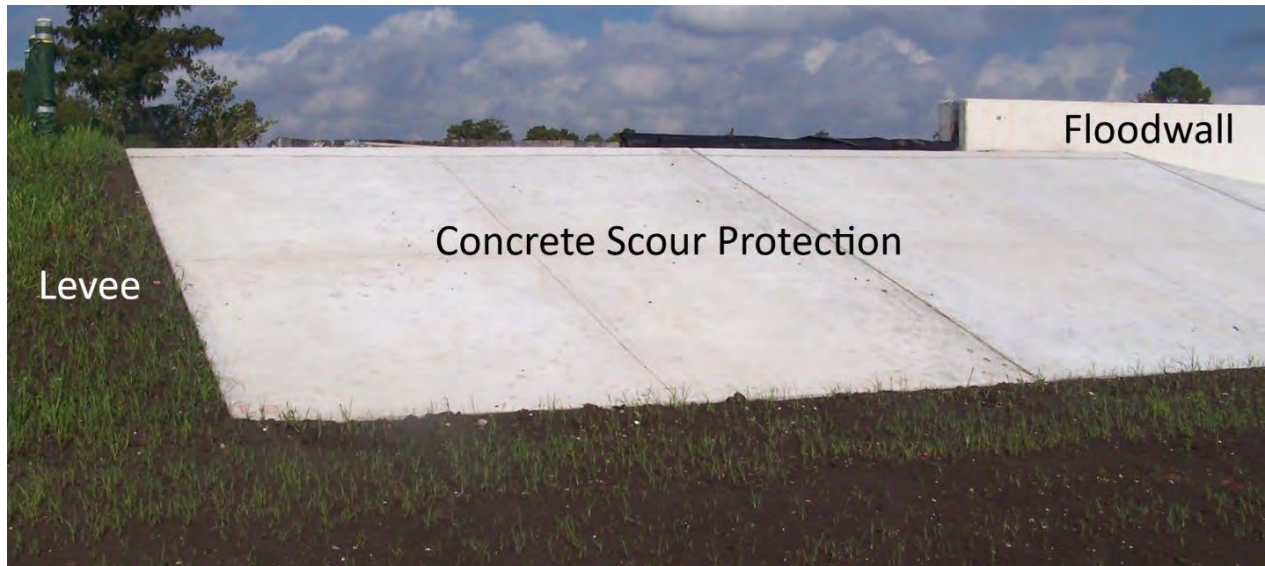
Figure 11: Illustration of Scour Protection at Levee-Floodwall Tie-in.
