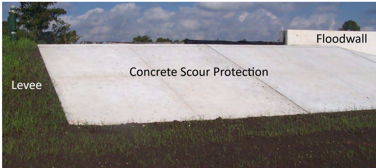
Figure 9: Concrete Scour Protection Example
