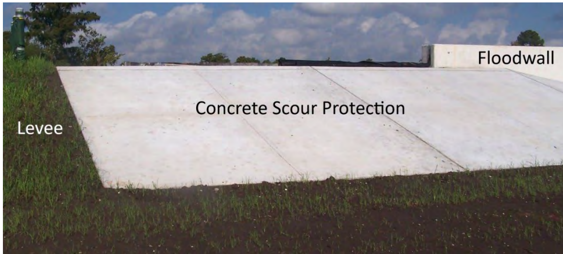
Figure 4: Concrete Scour Protection Example
