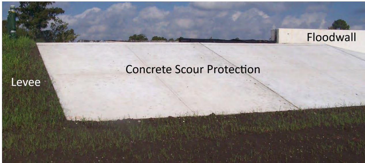
Figure 11: Illustration of Scour Protection at Levee-Floodwall Tie-in.
