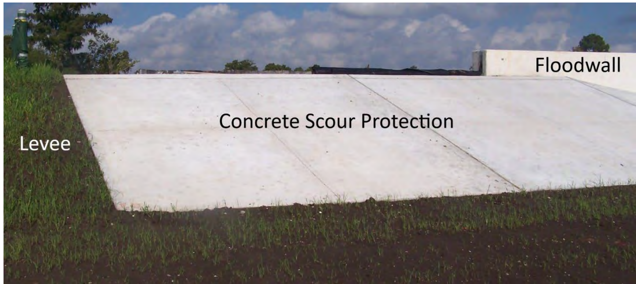
Figure 9: Illustration of Scour Protection at Levee-Floodwall Tie-in.
