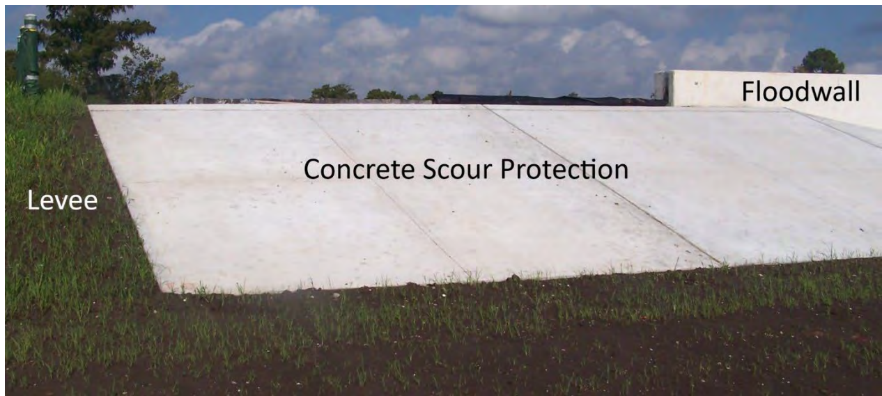
Figure 9: Concrete Scour Protection Example
