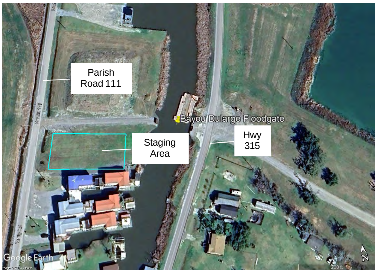
Figure 12: Staging and Access
