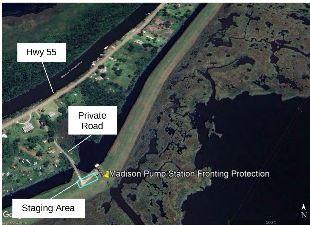
Figure 5: Access and Staging
