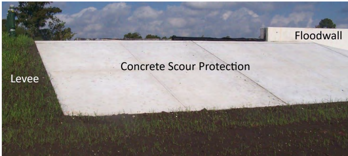
Figure 4: Concrete Scour Protection Example
