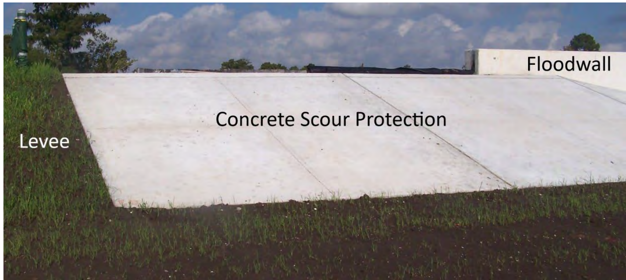
Figure 6: Concrete Scour Protection Example
