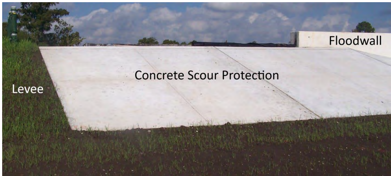
Figure 9: Illustration of Scour Protection at Levee-Floodwall Tie-in.
