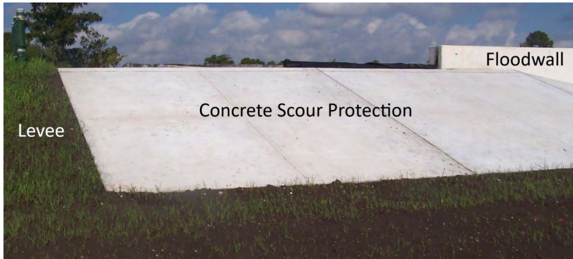
Figure 4: Concrete Scour Protection Example
