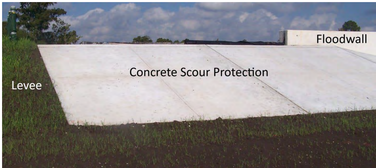
Figure 5: Concrete Scour Protection Example
