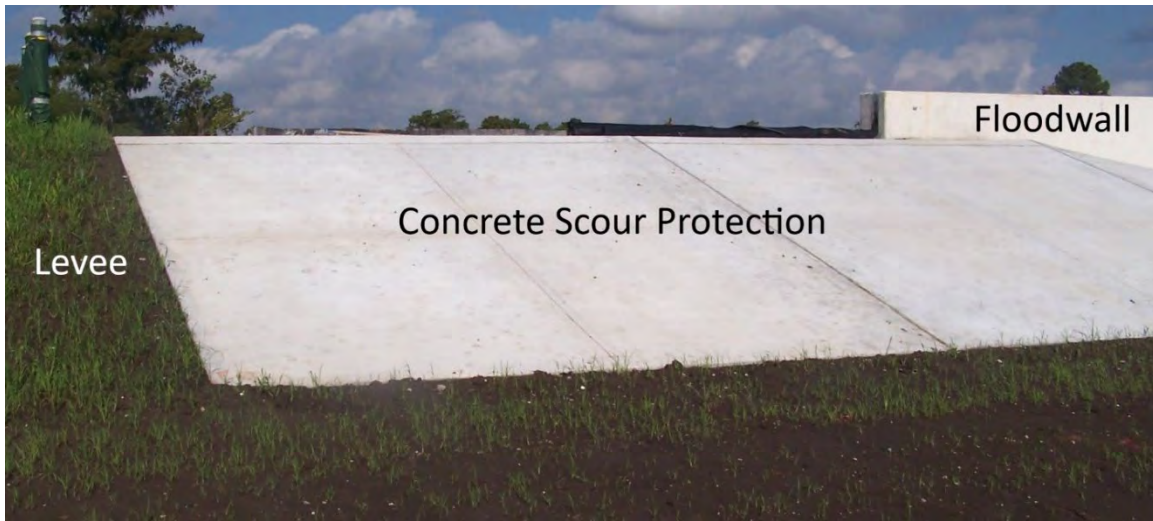
Figure 4. Concrete Scour Protection Example
