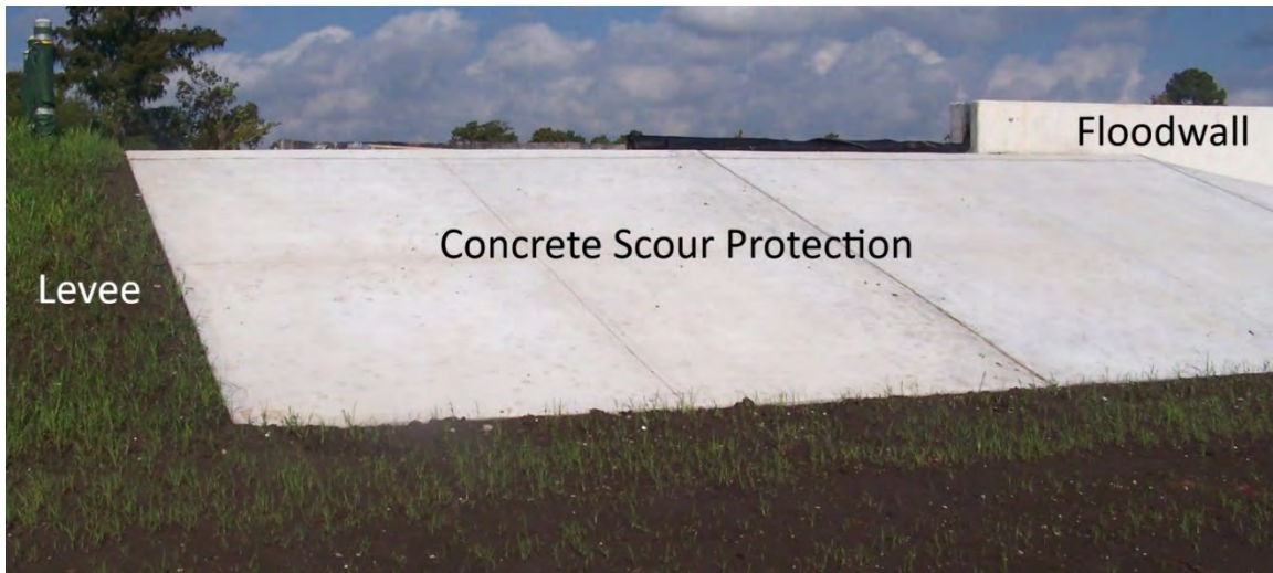
Figure 4: Concrete Scour Protection Example
