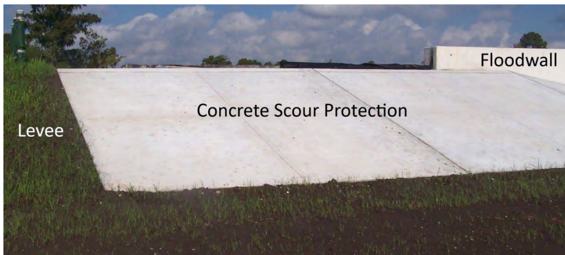
Figure 4: Concrete Scour Protection Example
