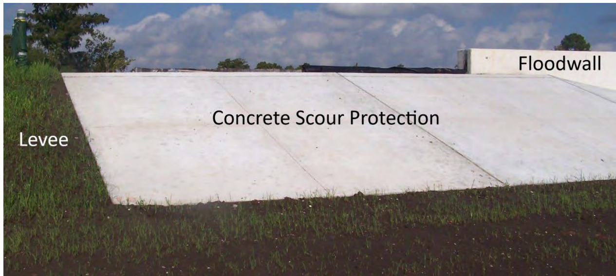
Figure 11: Illustration of Scour Protection at Levee-Floodwall Tie-in.
