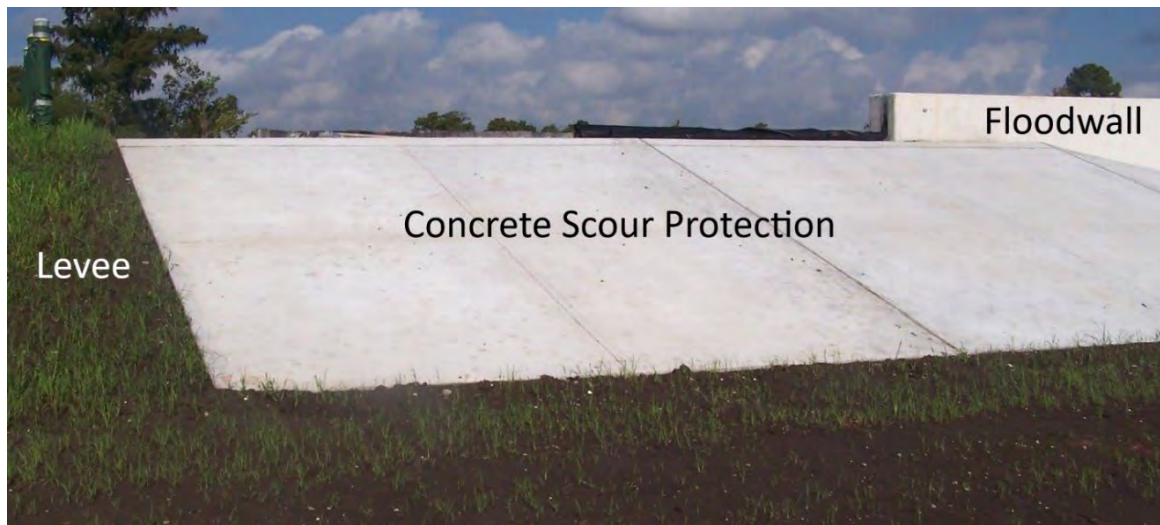
Figure 4: Concrete Scour Protection Example
